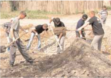
Road reconstruction in Voznesenskaya village, Ingushetia
