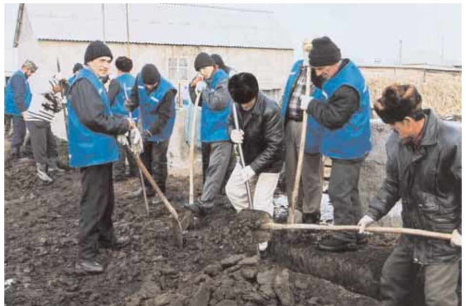
Digging a trench for water pipes in Kantyshevo village, Ingushetia
